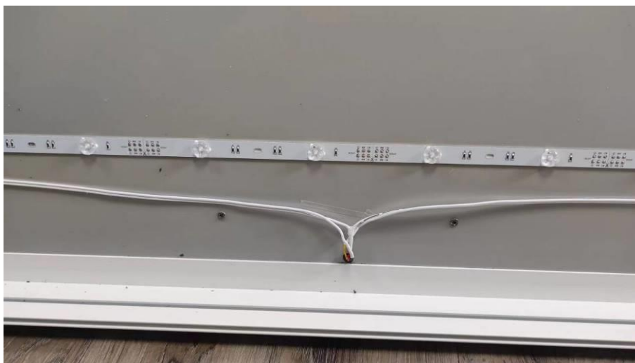
Internal view of CS-LBPR-CCT-960-24
